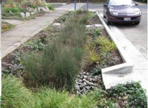
garden is a planted bed that allows rainwater runoff from impermeable urban areas to be absorbed.
